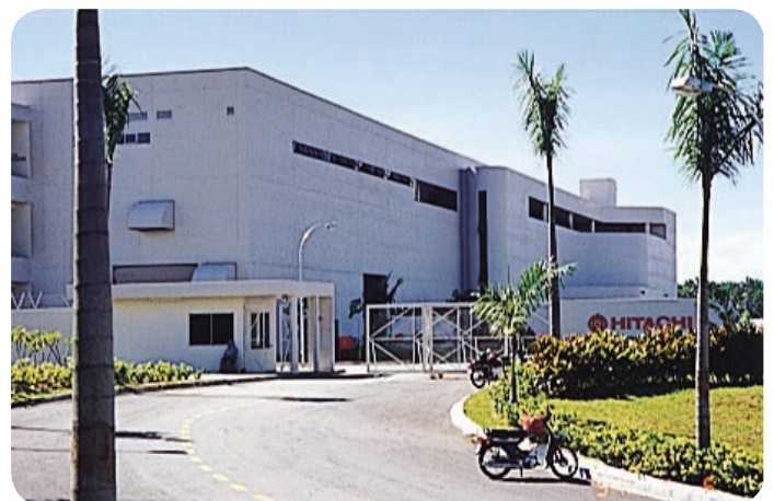
Hitachi Air Conditioning Products (M) HAPM works, Malaysia
