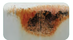
Normal cabinet material after 600 hours
